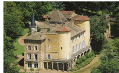
Saint Point Château Lamartine 100 kW
